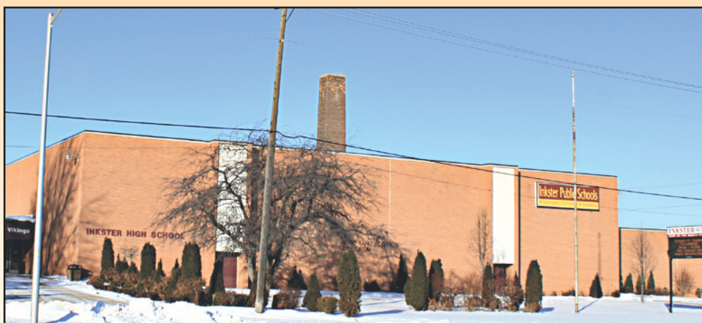
Inkster High School, built in 1952, will be demolished by order of the Wayne County Regional Educational Service Agency.
