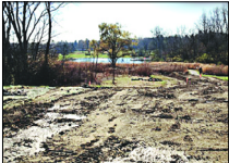
Construction of a 75-foot circular swale which will contain rainwater and runoff from the 200-space parking lot in McCumpia Park is under way. Photo by Don Howard
