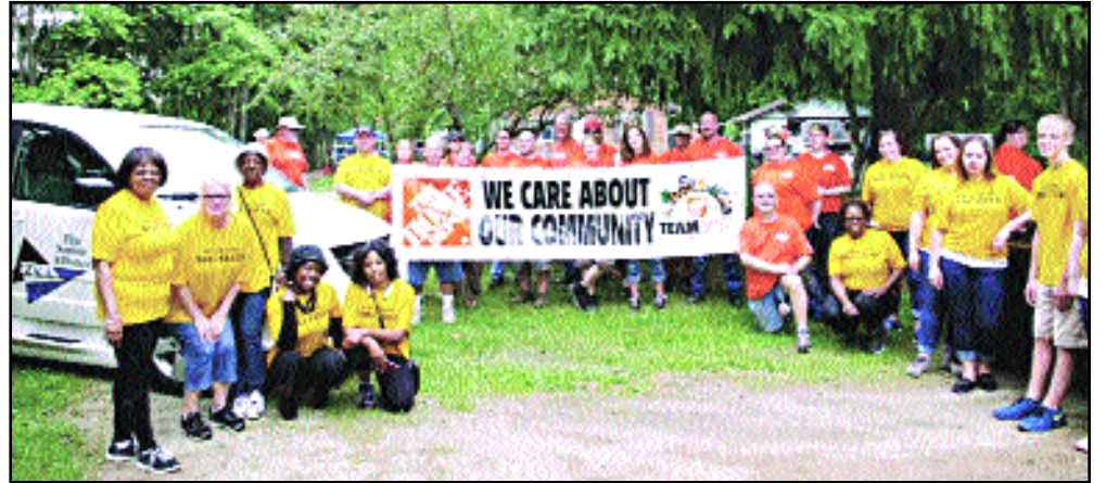
Nearly 50 volunteers from Home Depot and The Senior Alliance worked to renovate and repair the home of a World War II veteran in Van Buren Township early this month. The Plymouth Home Depot was the host store for the project. Photo by David Wilson
