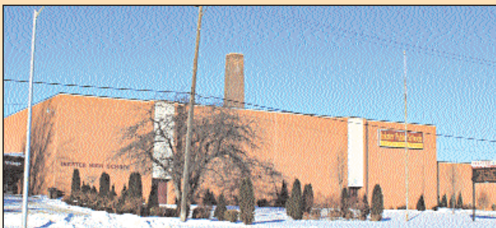
Inkster High School, built in 1952, will be demolished by order of the Wayne County Regional Educational Service Agency.
